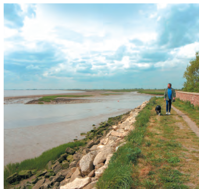
Flood defence at Brough
